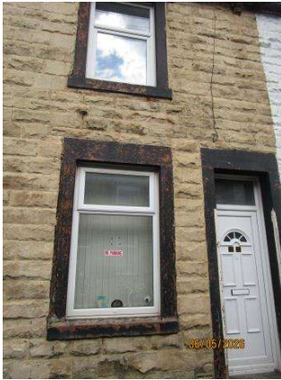
Photo showing the front elevation at the time of the audit
