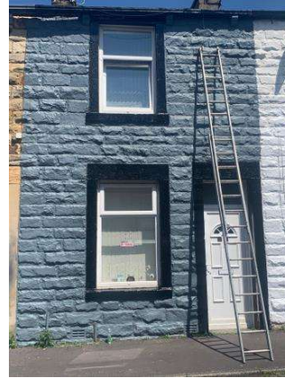
Photo showing the work completed at the post audit
