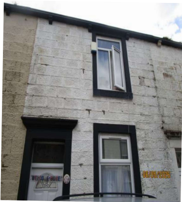
Photo showing the front elevation at the time of the audit
