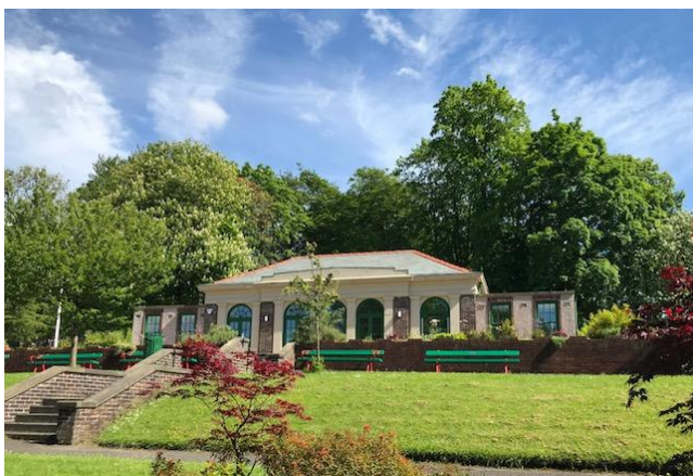
Pavilion exterior following restoration
