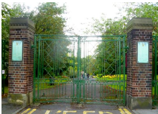
Old gates before restoration
