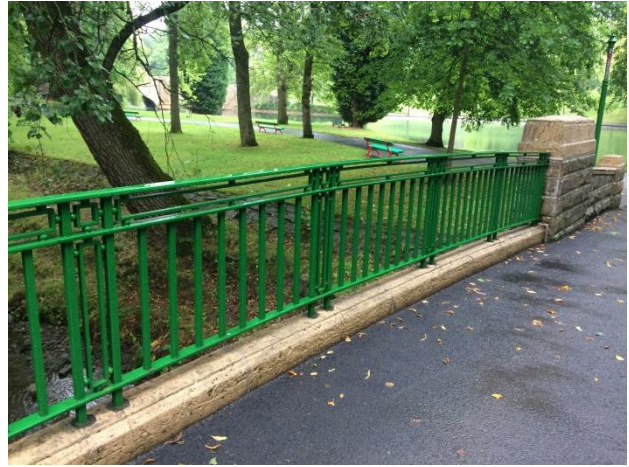
Lower bridge with new parapet railings
