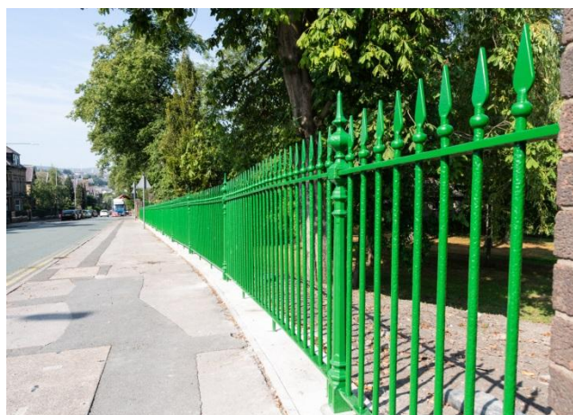
New railings after restoration
