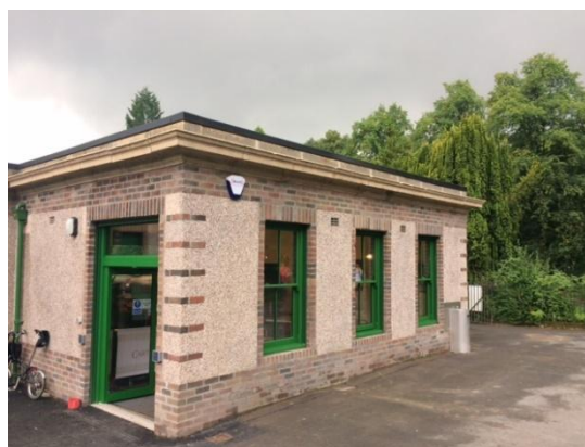
The Boat House following conversion to a cafe
