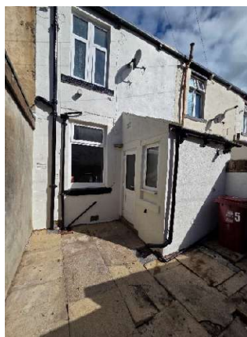
Rear elevation after work completed
