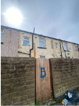
Rear elevation on audit day
