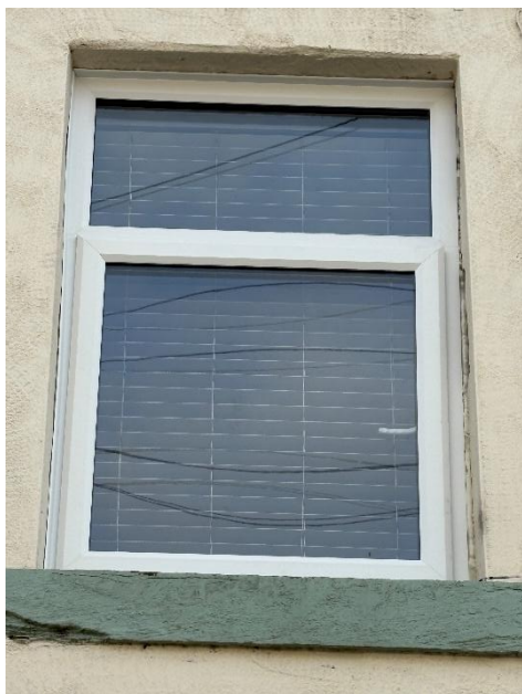
New escape window fitted
