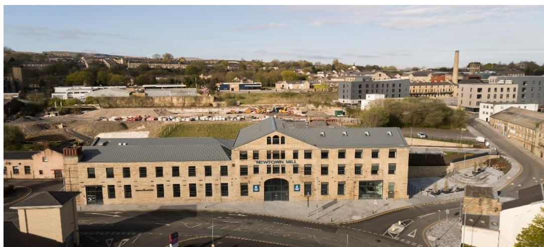
The redeveloped Newtown Mill, Queens Lancashire Way, Burnley (Source: BBC)
