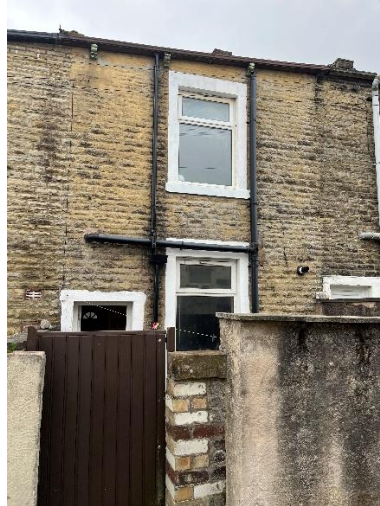
New rear timber gate fitted
