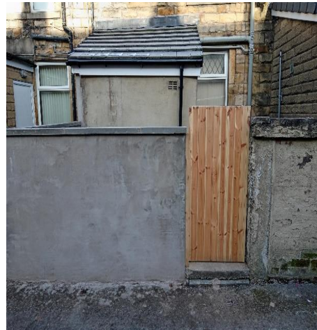
Yard wall demolished and rebuilt
