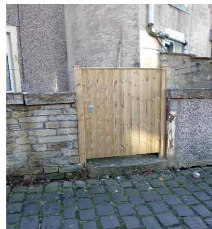
New gate fitted
