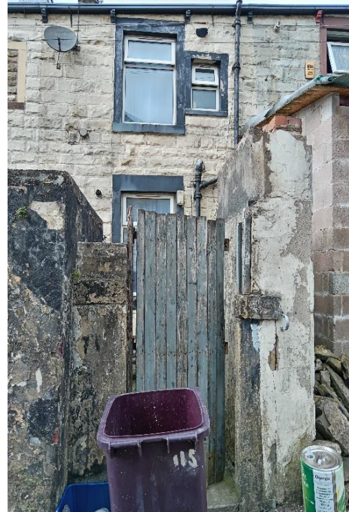
All windows reglazed in 48 hours and made secure
