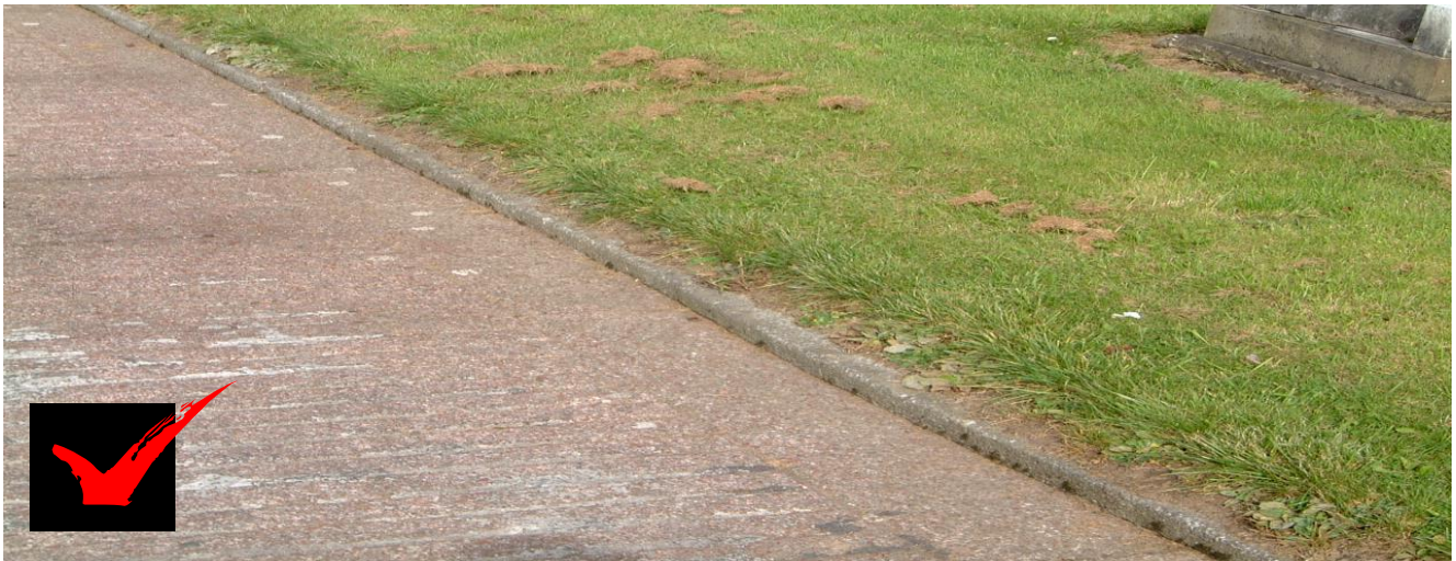
75mm spray width produces correct result
