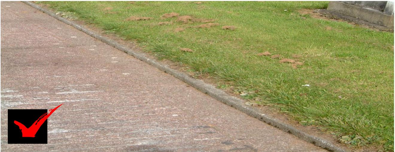
**75mm spray width produces correct result**
